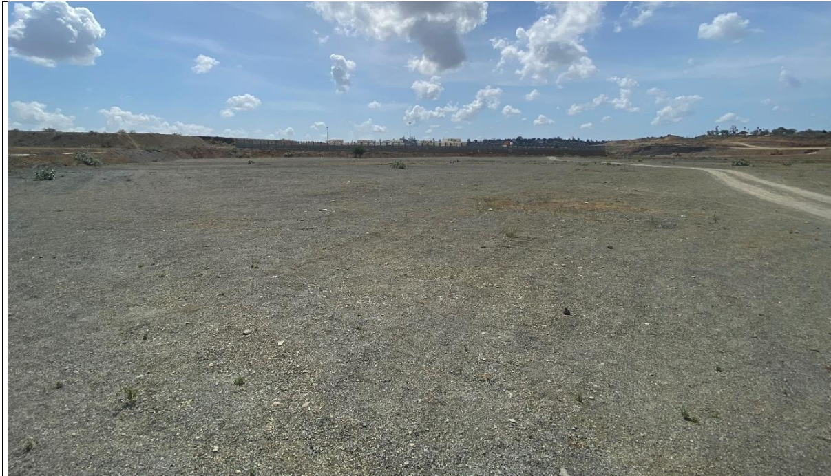
Figure 6.8 Project Site sowing land clearance and grading
